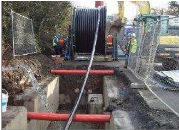
Figure 8.9: HV Cable Pulling Procedure (Typical Drum Setup)
