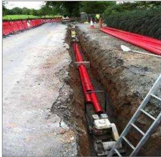
Figure 8.1: Typical 110 kV Underground Duct Installation
