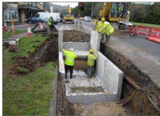
Figure 8.8: Typical Joint Bay under Construction (Pre-Cast)
