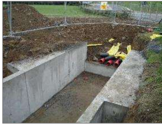
Figure 8.7: Completed Joint Bay prior to Cable Installation (in-situ)
