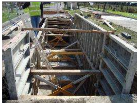
Figure 8.6: Typical Joint Bay under Construction (In Situ)
